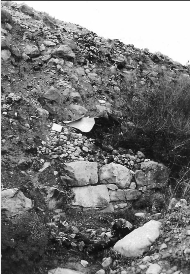
Photo 1. View of the Mycenaean dam with remnants of the eastern retaining Cyclopean walls on the side of the active channel. The core fill is made of dirt and large limestone blocks.
